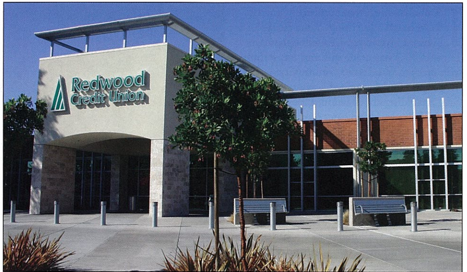
Redwood Credit Union's corporate offices in Santa Rosa
